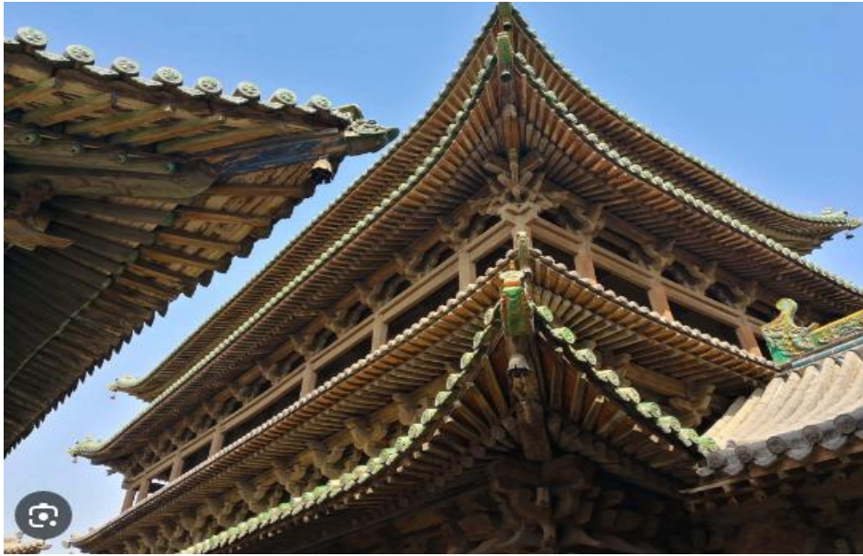
Figure 8. Traditional Roof Style in Chengdu [Source: Lily Sun China Tours (n.d.)]
