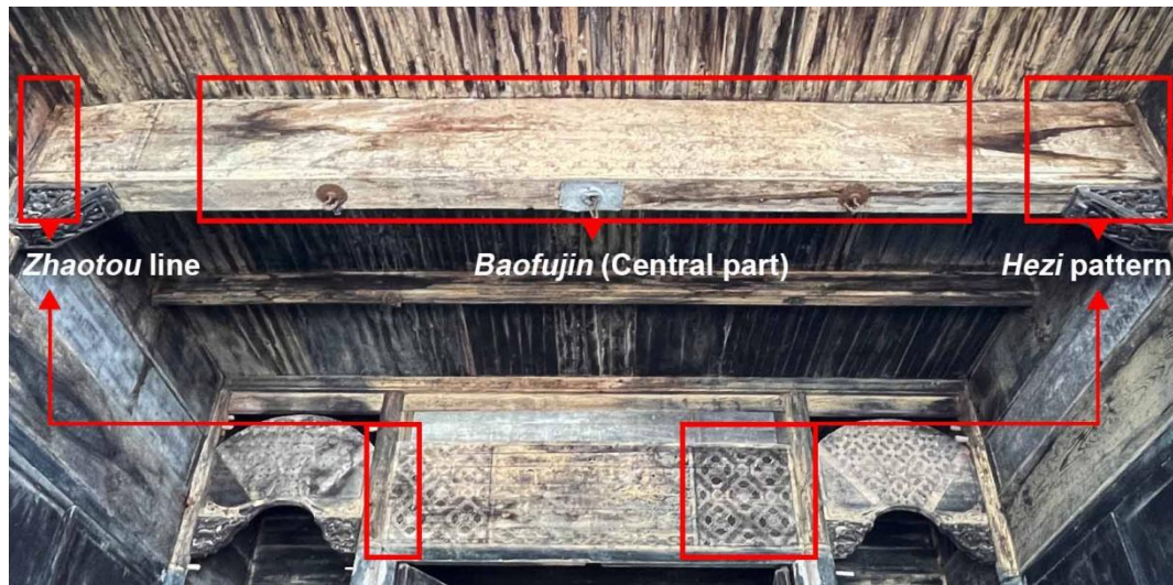
Figure 9. Segment Composition—The Composition of the Baofujin Color Painting Containing the Zhaotou Line and Hezi Patterns (Source: Photographs and design by the author)
