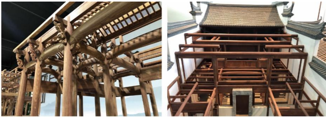
Figure 2. Cheshang Mingzao Architectural Structure: The Practice of Exposing the Wooden Beam System in the Interior of Huizhou Buildings (Source: Photographs by the author in Huizhou Jixi Museum)
