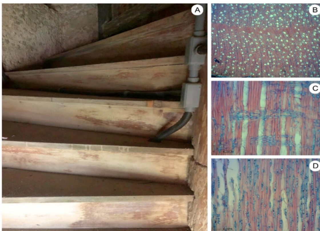
Figure 5. Constructive element and respective wood anatomy of Aspidosperma sp. (Apocynaceae), Nossa Senhora da Graça Church, São Francisco do Sul, Santa Catarina State, Southern Brazil. Caption: (A) Bell tower staircase steps. (B) Transverse section. (C) Radial longitudinal section. (D) Tangential longitudinal section.
