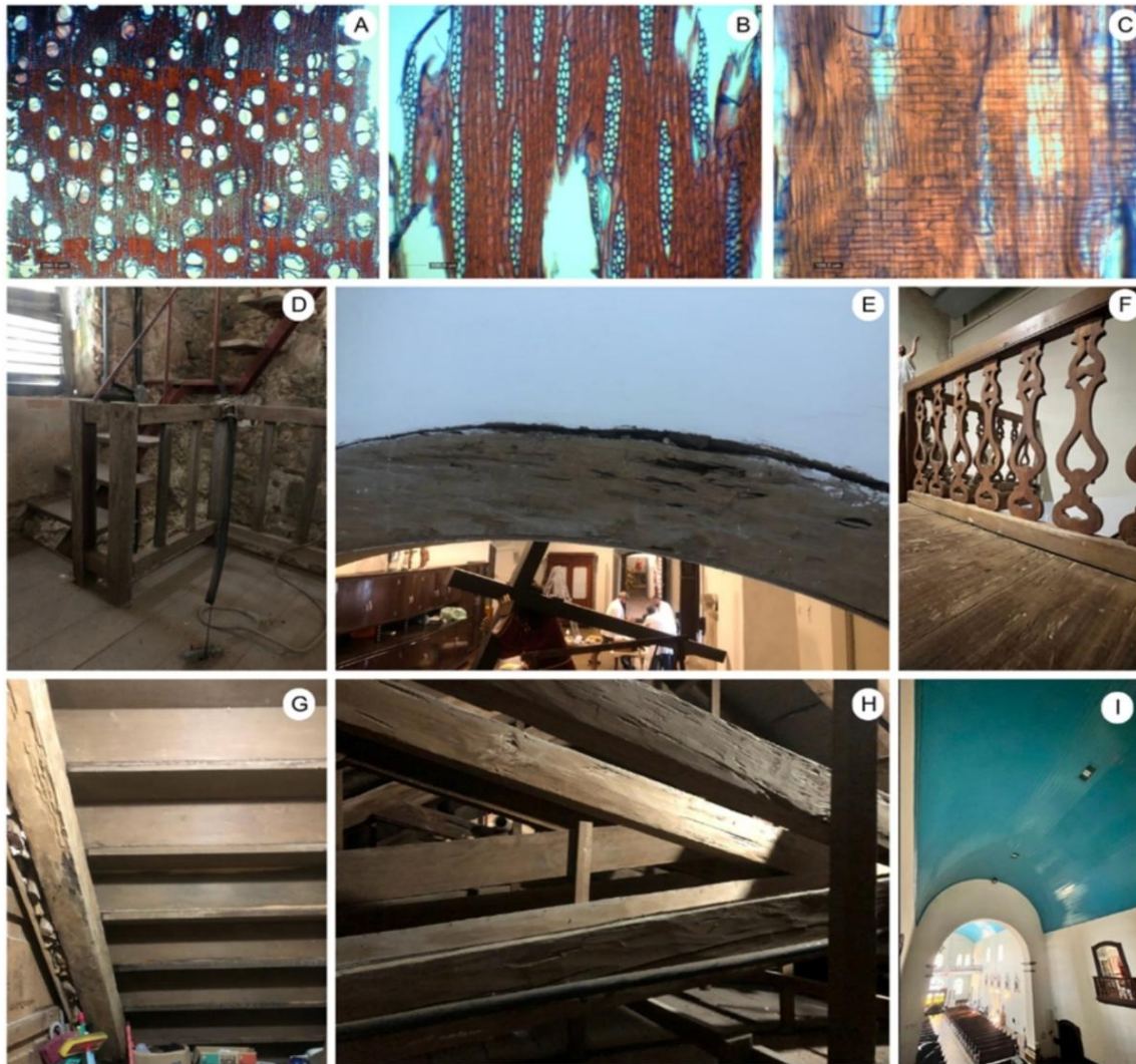
Figure 10. Constructive element and respective wood anatomy of Ocotea porosa (Lauraceae), Nossa Senhora da Graça Church, São Francisco do Sul, Santa Catarina State, Southern Brazil. Caption: (A) Transverse section. (B) Radial longitudinal section. (C) Tangential longitudinal section. (D) Bell tower railing. (E) Sacristy access frame. (F) Baluster of the museum railing. (G) Step below the sacristy staircase. (H) Roof truss (old piece). (I) Roof lining.
